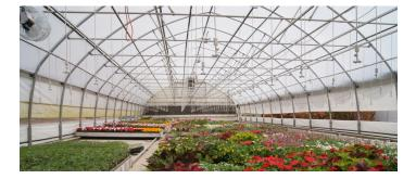
The North Slope is designed to shed snow and allow maximum light into the greenhouse for Northern climates. We have found that its generous Gothic peak makes it easy to cool with natural ventilation so that it excels in mild to hot climates as well. The North Slope is a commercial grade quonset / high tunnel greenhouse. The North Slope's Gothic arch design with no flat spots is stronger and drips less.
